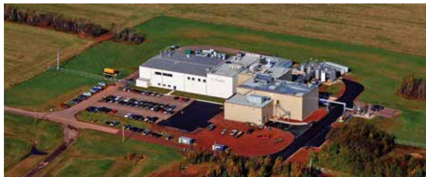
Photo 1: BioVectra's API manufacturing facility
